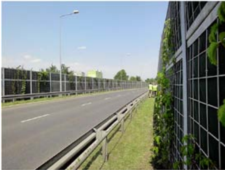
Photo 3 — Sound barriers on DK 79 in the town of Jaworzno
