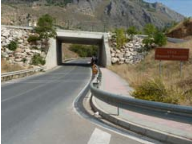
Photo 1 — New bridge in the town of Loja (ES) that resolved the road-level railway crossing problem and reduced the accident rate to zero.
